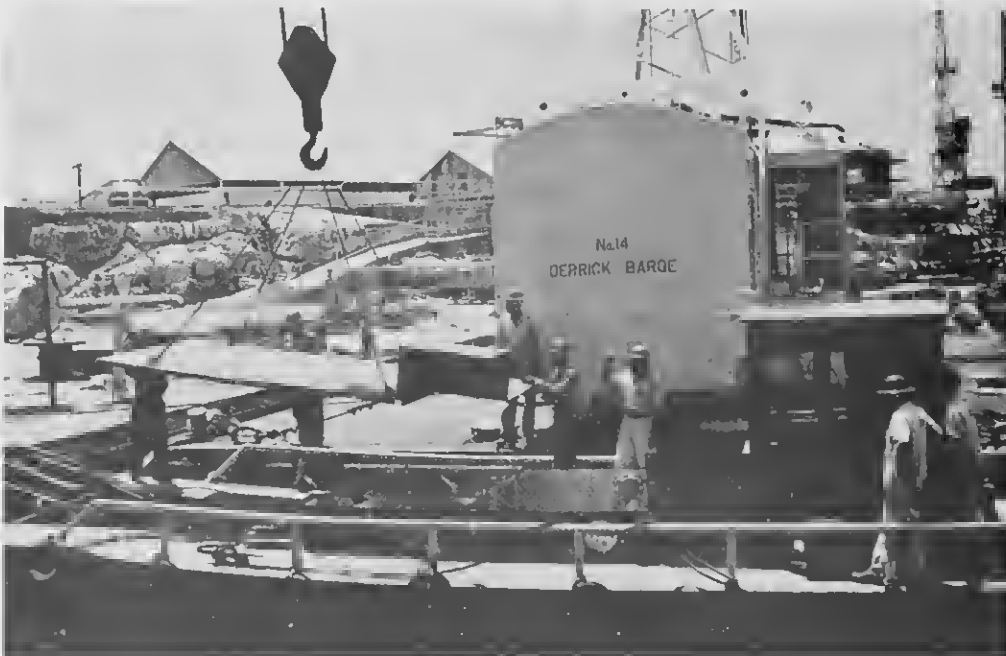
BY FITTING this steel plate over the engine compartment, the fire boat can be quickly converted into a work boat when needed. The boat resulted from tremendous cooperation among Marine, TSD and Mechanical personnel.
